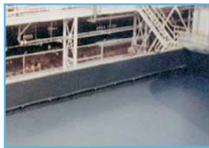
Bund after relining
